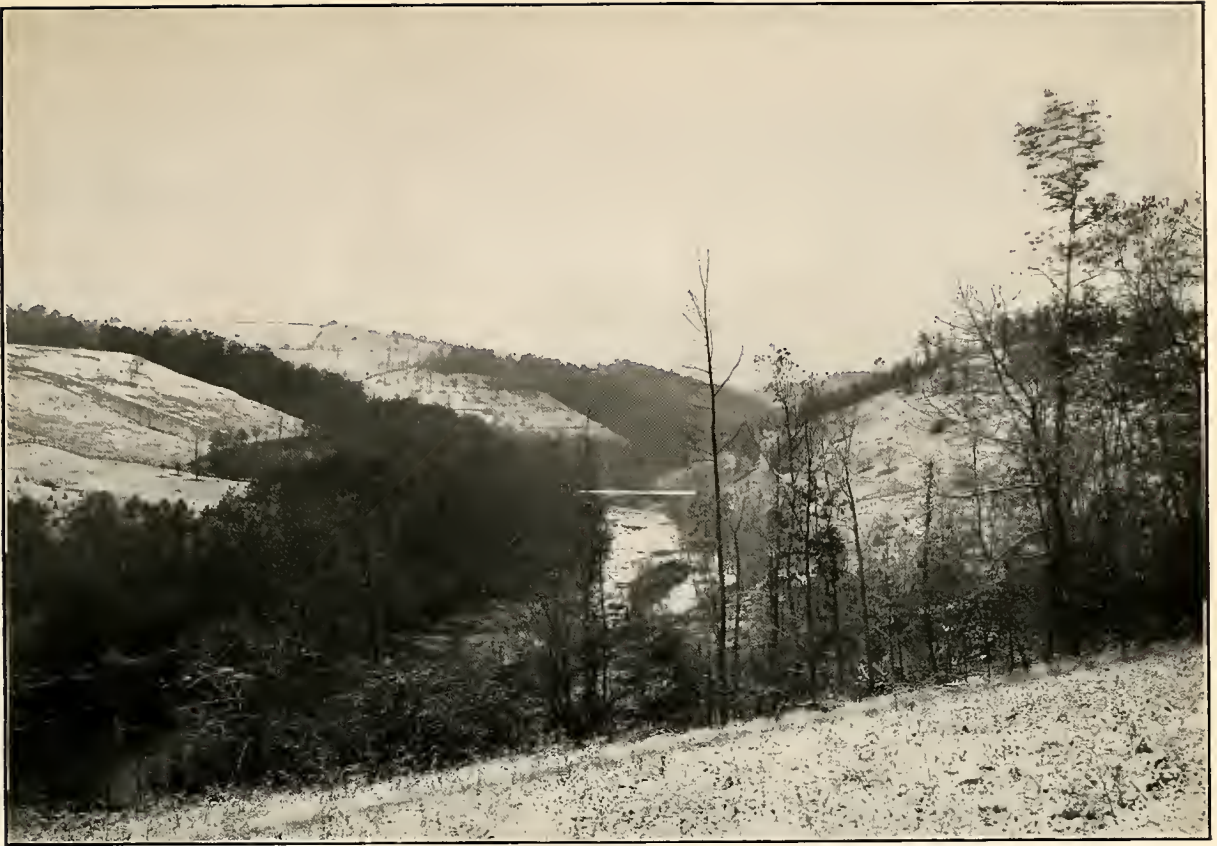
BUCKHANNON RIVER, W. VA., NOVEMBER, 1910. View up stream, showing crest of proposed dam.
